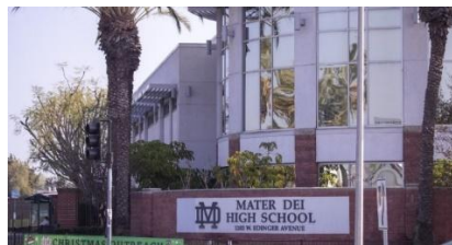
Mater Dei High School, Los Angeles, California
